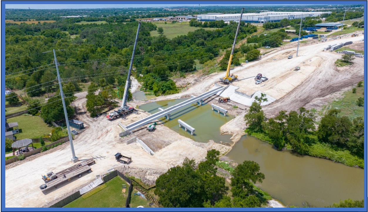
Beam Setting on Old Settlers Boulevard Extension looking Southwest towards Red Bud Road, June 2025
