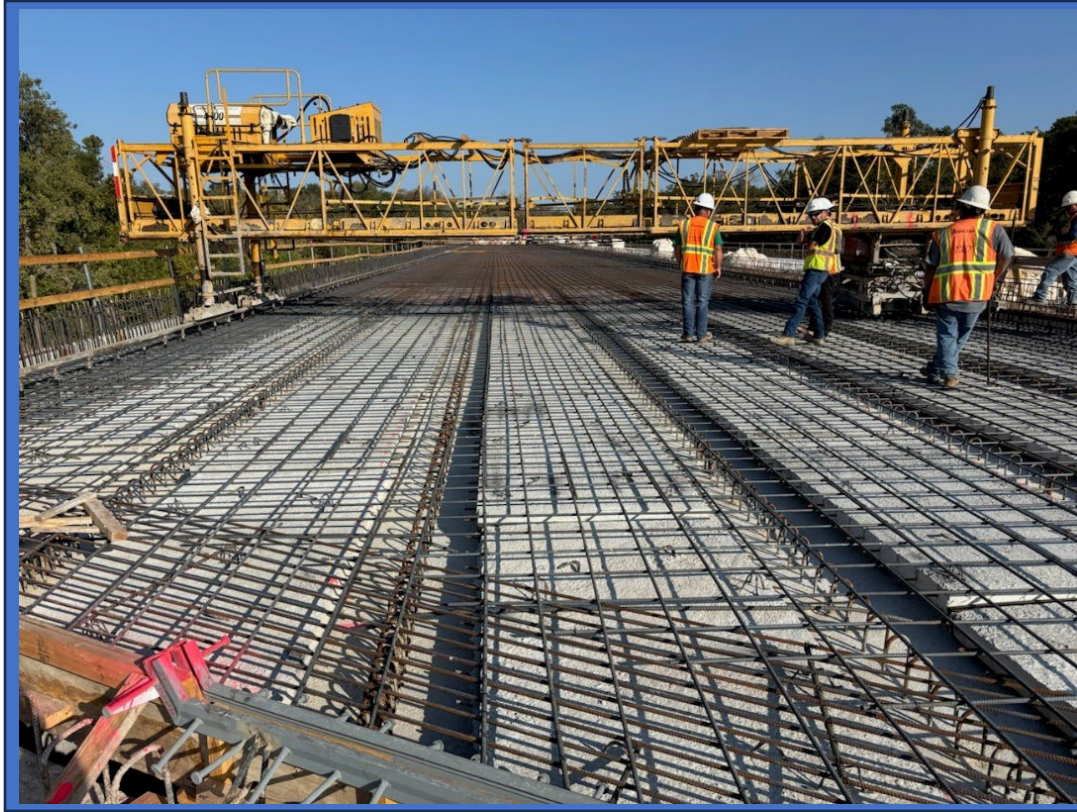
Bridge Deck on Wyoming Springs Extension concret preparation
