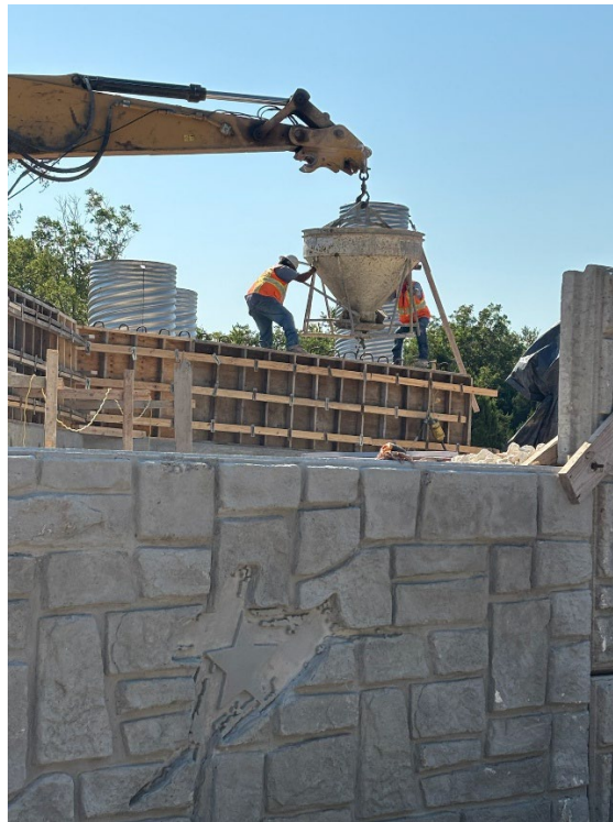
Bridge Deck on Wyoming Springs Extension concret application
