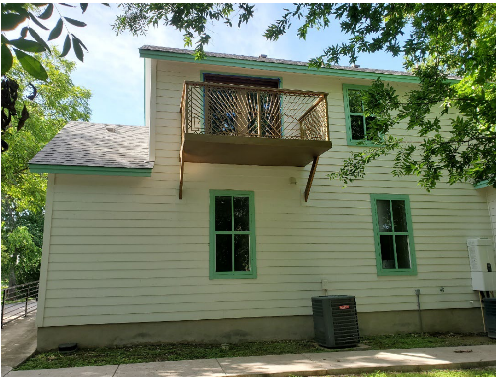
June 2026 photo of new balcony. The balcony doors have grilles similar to the west doors. Photo also shows the new, lighter-weight screens, and unscreened mechanical equipment.
