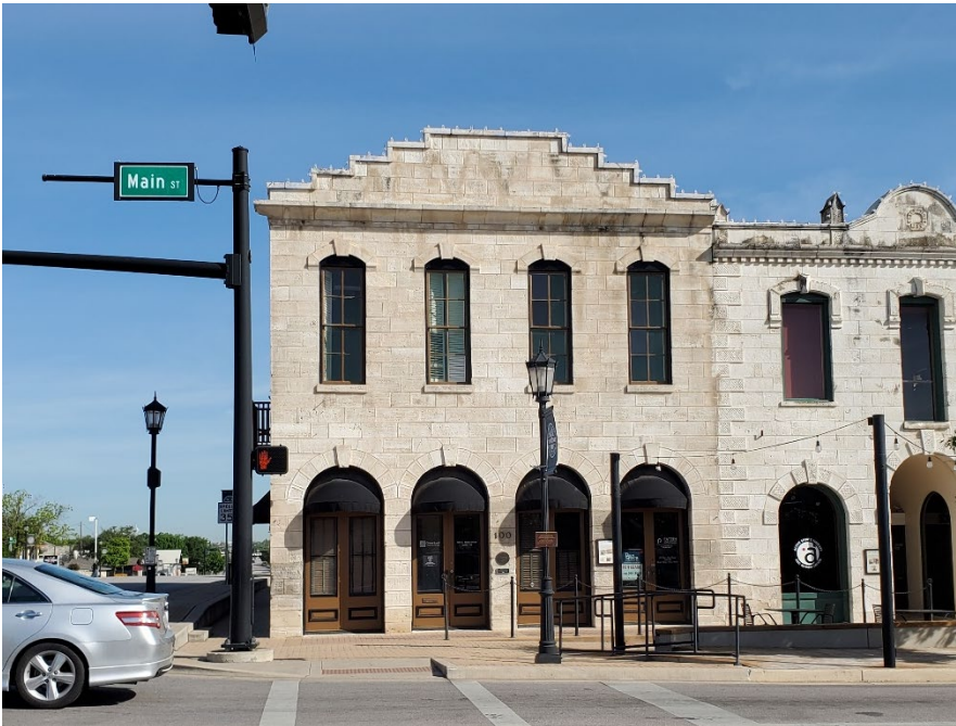
2024 photo, south (front) side
