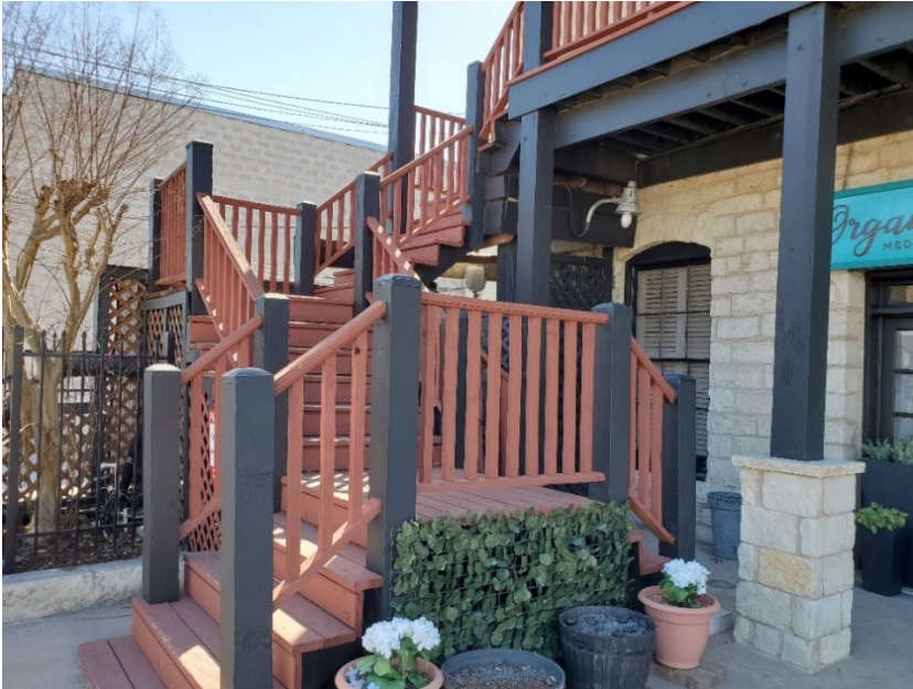
Previous back staircase (2022 photo)
