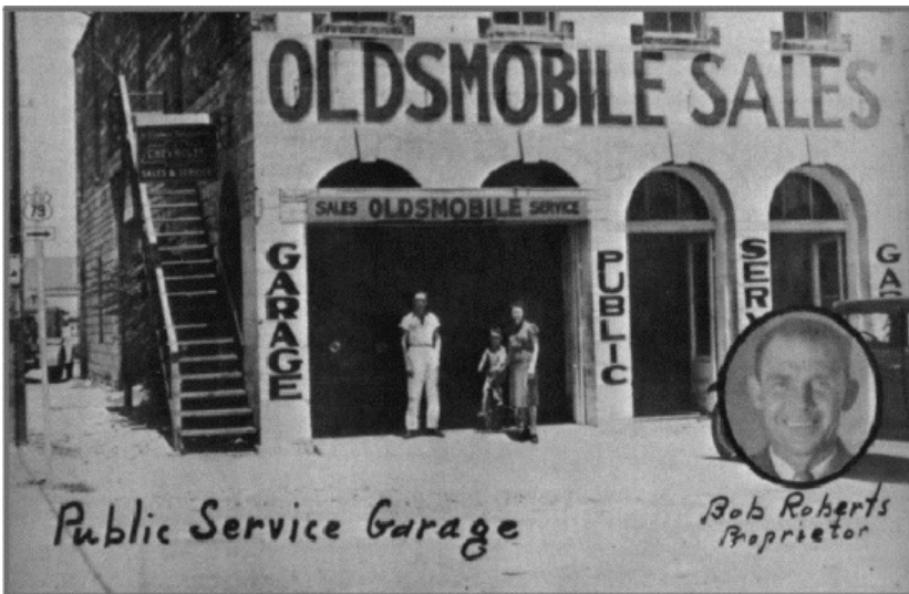
1938 photo showing alterations for vehicle access
