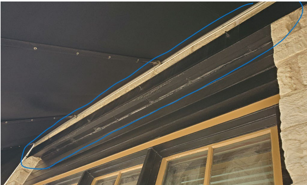
Photo of west lintel under awning, November 2024
