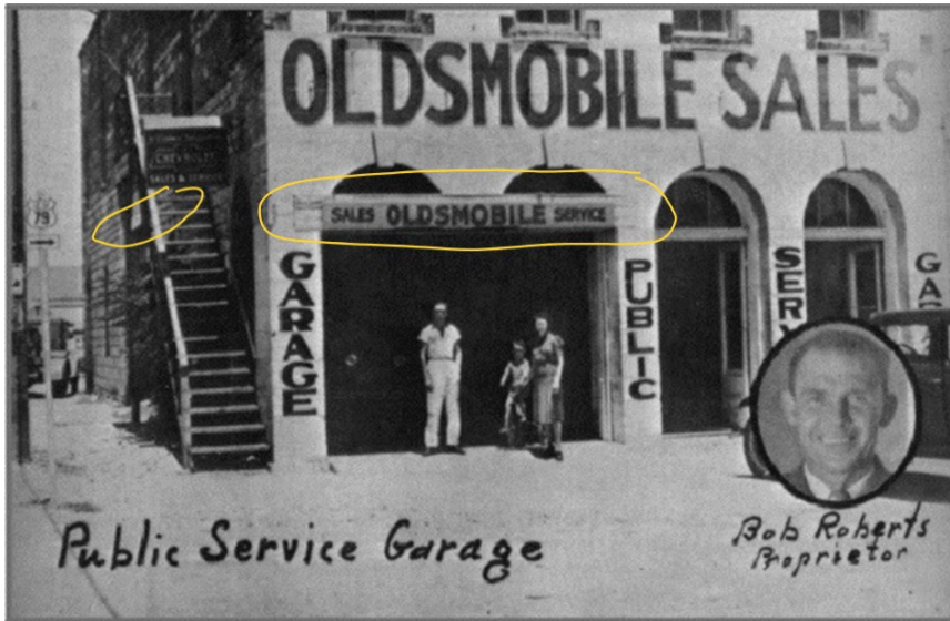
1938 photo indicating lintels
