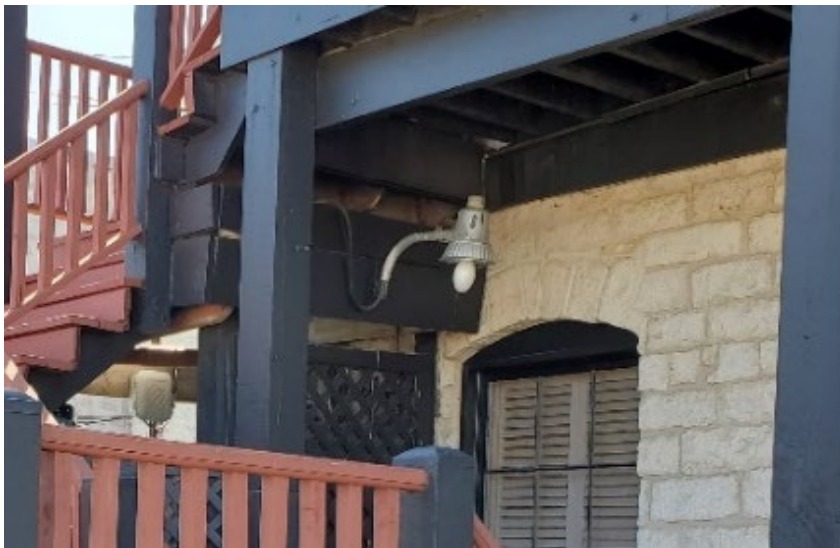
Current light fixture (2022 photo)
