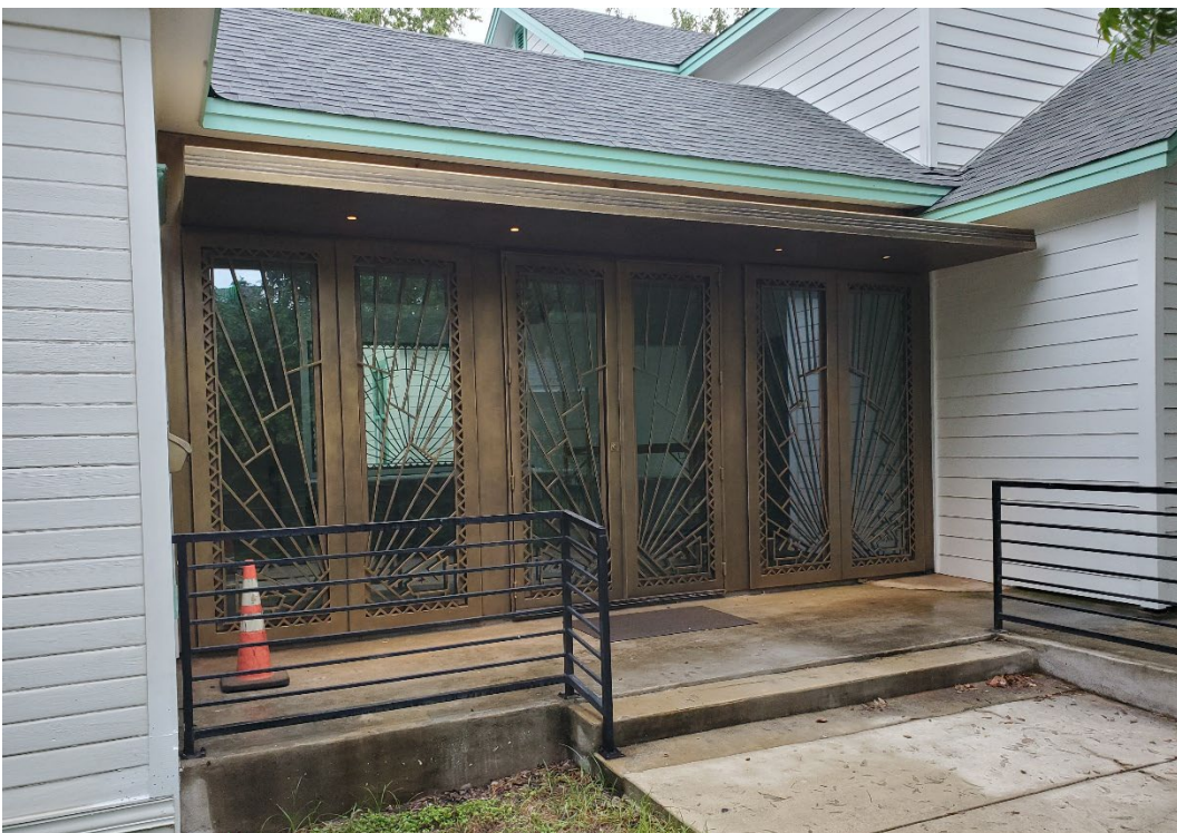
June 2026, showing new doors and canopy.
