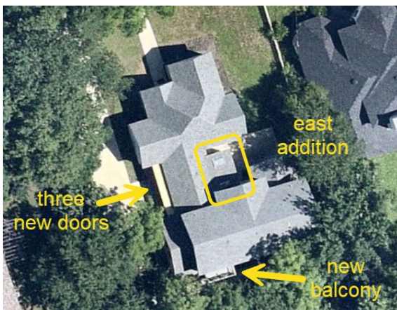
2026 aerial photo indicating locations of different parts of the project.
