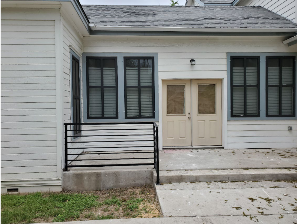
2023 photo showing the first set of screens
