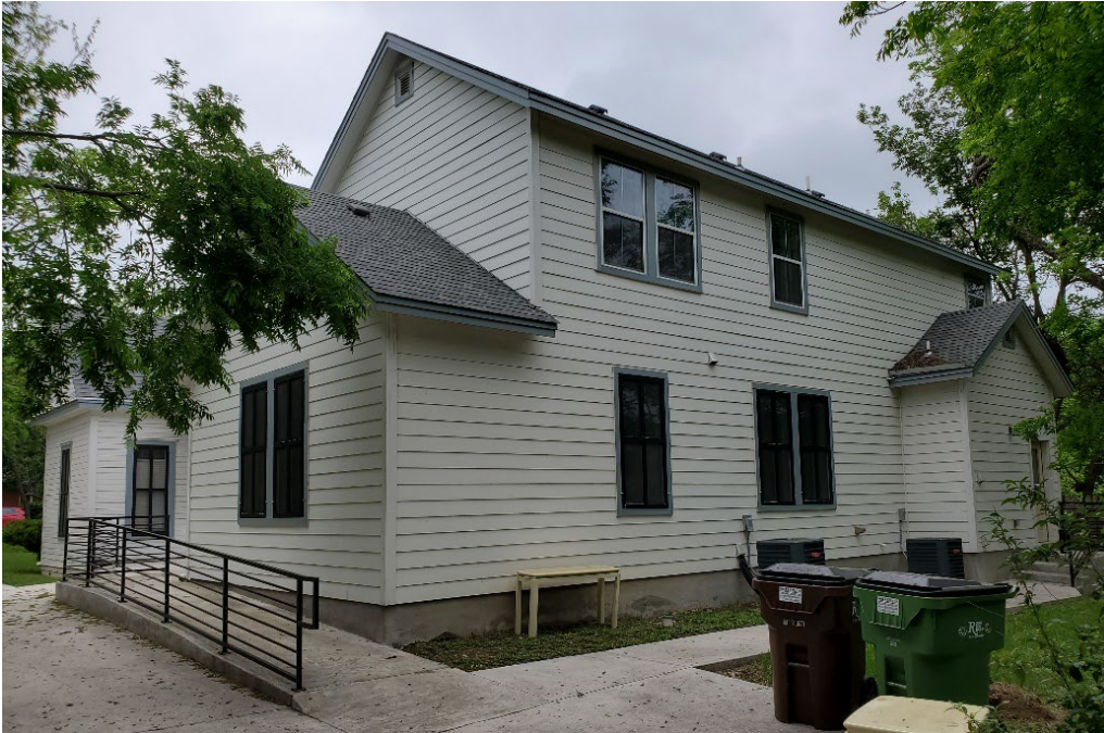
2023 inspection photo. The older set of screens is in place.
