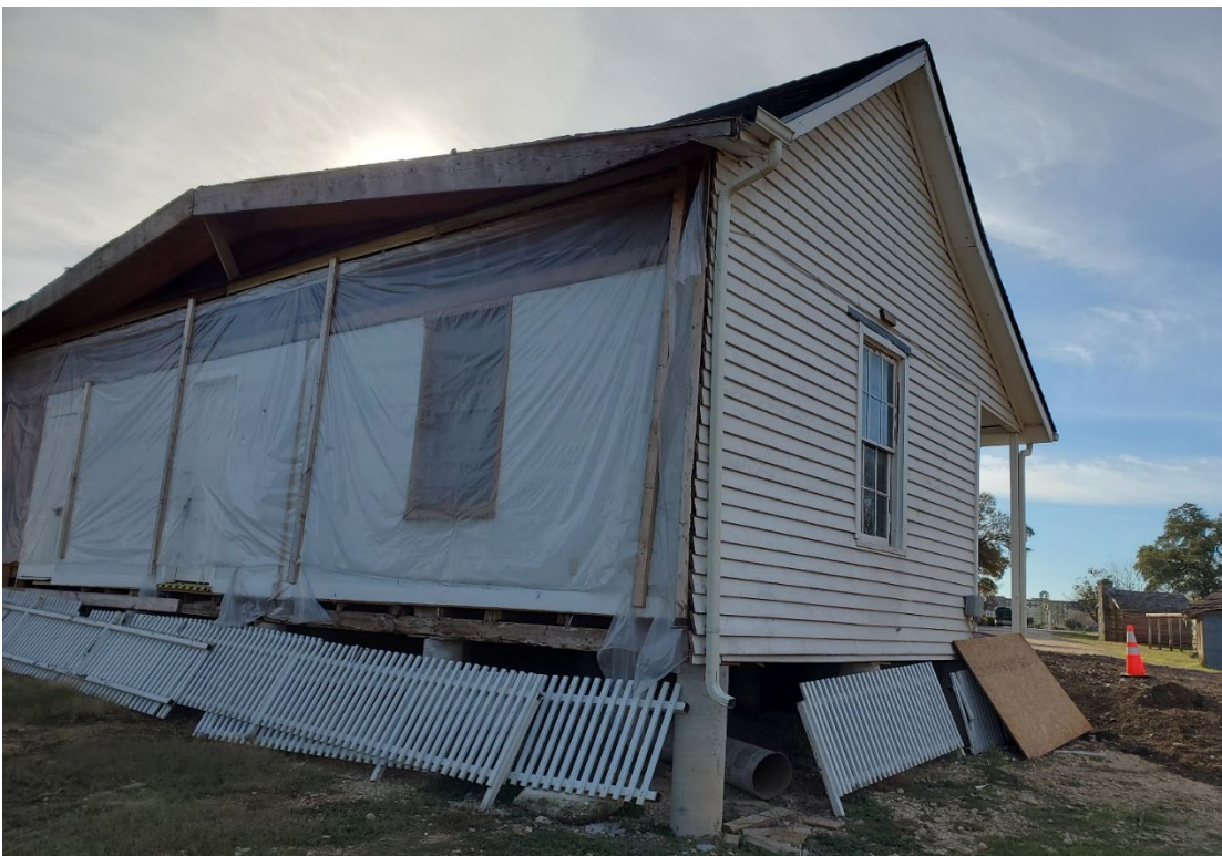
The Palm House at the Old Settlers Association, north (back) side. The Round Rock Chamber was attached to the back wall, currently protected with plastic sheeting. The remains of the roof cricket will be removed and the eaves extended backward.
