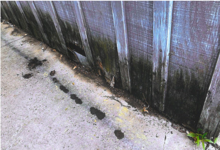
Detail of water-damaged siding on north wall
