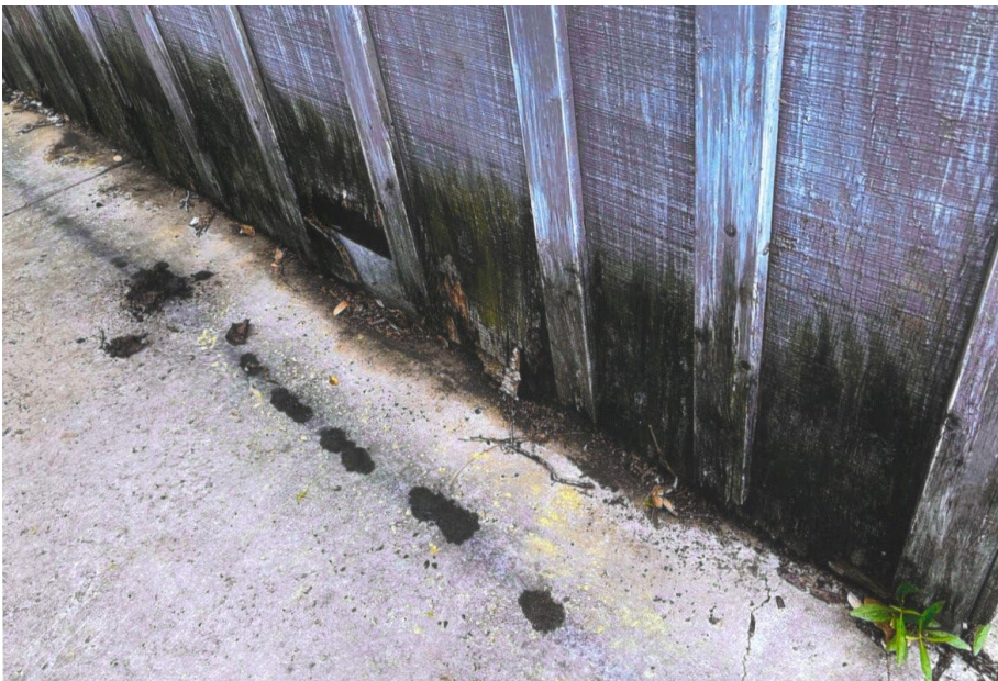
Detail of water-damaged siding on north wall
