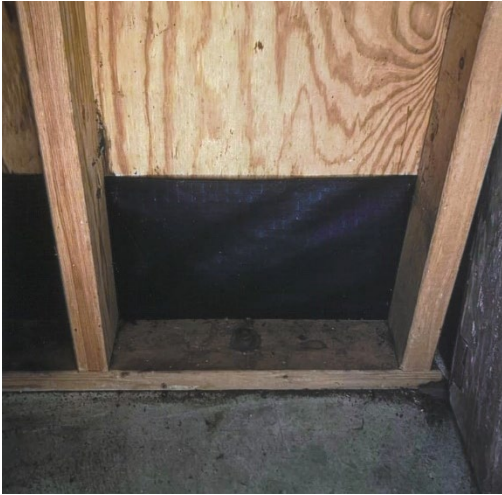
Detail of interior; framing is protected from moisture and damage is confined to the sheathing.
